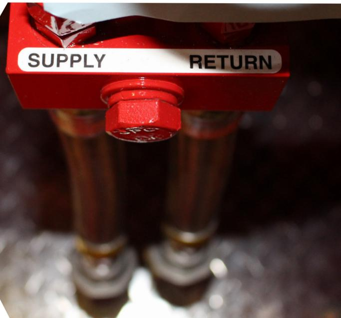
Fuel is one of the 3 key components to make your diesel fire pump driver run. The engine must be equipped with quality fuel hoses used to isolate engine vibration from the fuel lines and fuel tank. These hoses are essential to provide enough fuel to power the engine while having the ability to stand up against wear and tear of regular usage and corrosive environments.
